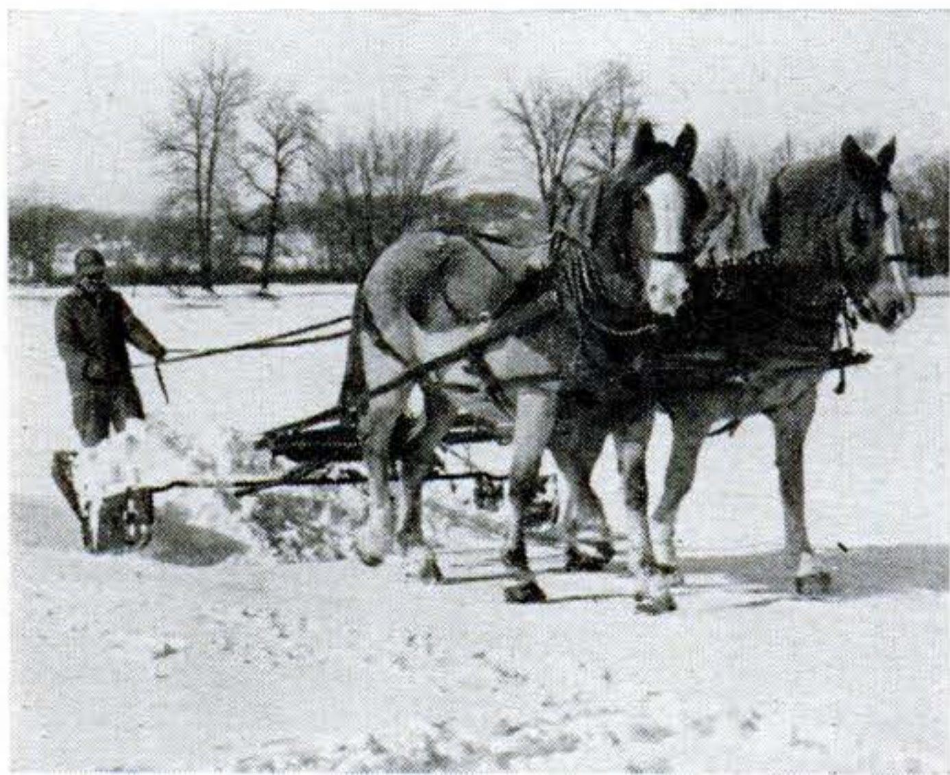
2. Horse-drawn scrapers are first on the job, cleaning snow off the ice. The sheet must be frozen to a thickness of at least 12 inches before the harvesting operation can begin.
